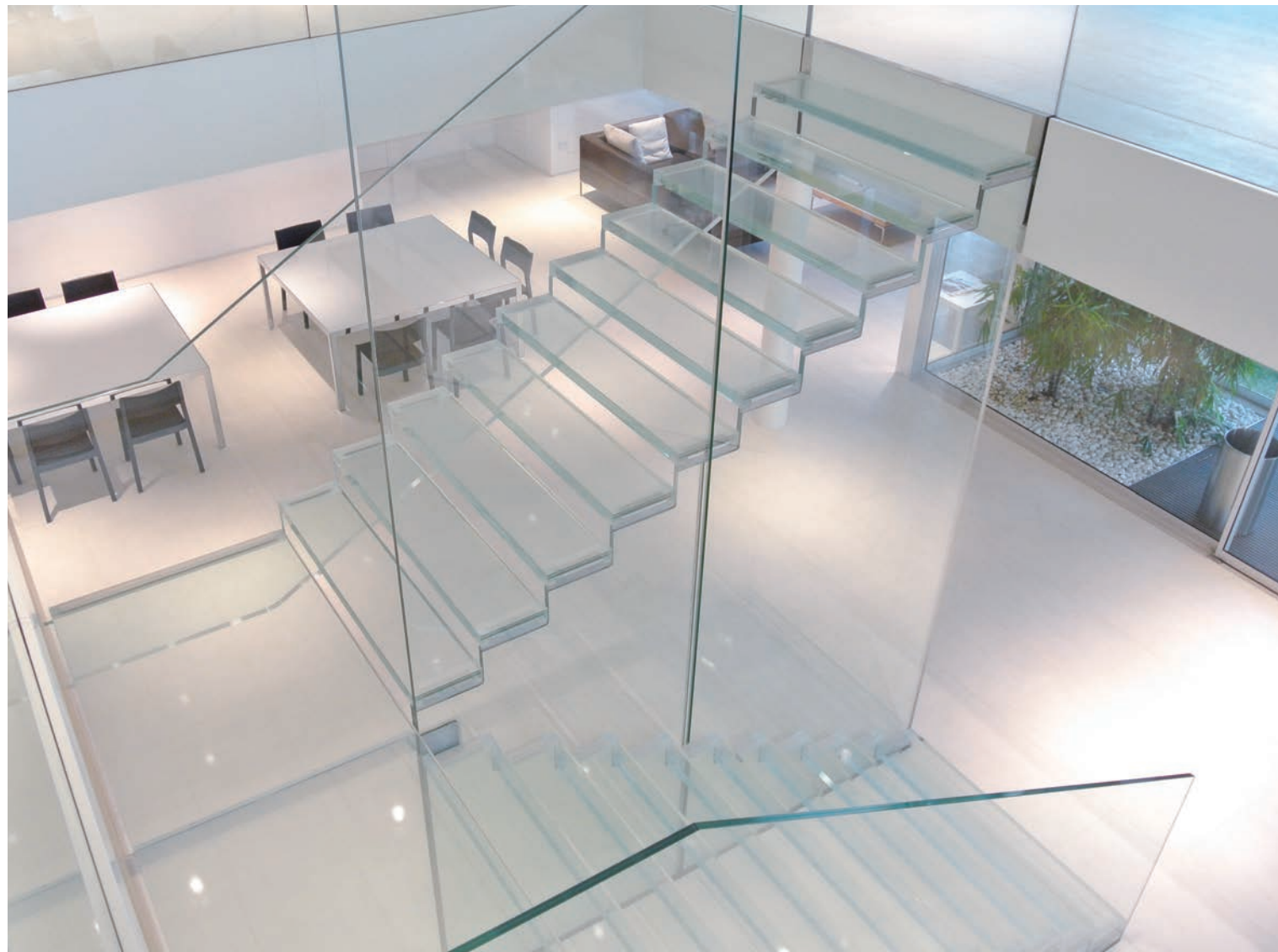
/ Pixel Flooring Self-supporting glass staircase Glass structure project: Michel Palumbo Eng. Vetrostrutturale® Architectural project: Studio Monica Armani
