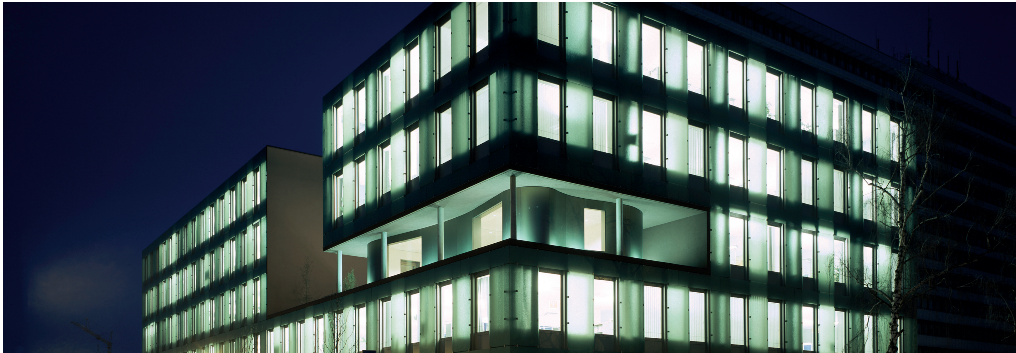
/ Silk Glass façade translucent cladding, Siemens Building, Erlangen/DE
